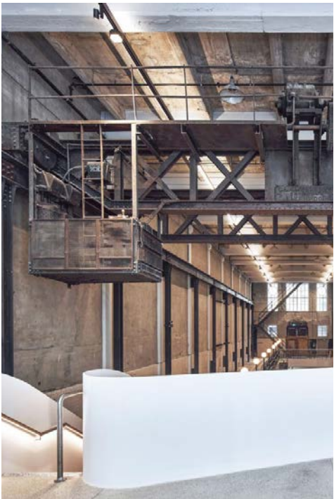
Substation No. 164, Sydney Timber flooring was repurposed into formwork for concrete floor slab as well as wall panelling in the interiors.
